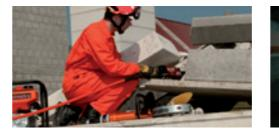
A perfect combination: crushing concrete with the CC 23 and cutting re-bar with mini cutter CU 4007 C or SMC 5006.
